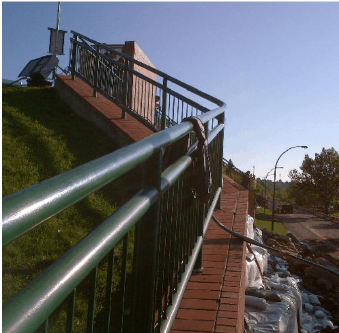
AESRD Temporary Station – Medicine Hat 2013
