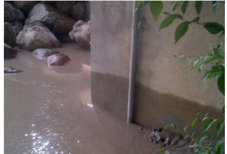
Medicine Hat WSC shack: High water mark and 5500 m 3 /s predicted level est.
